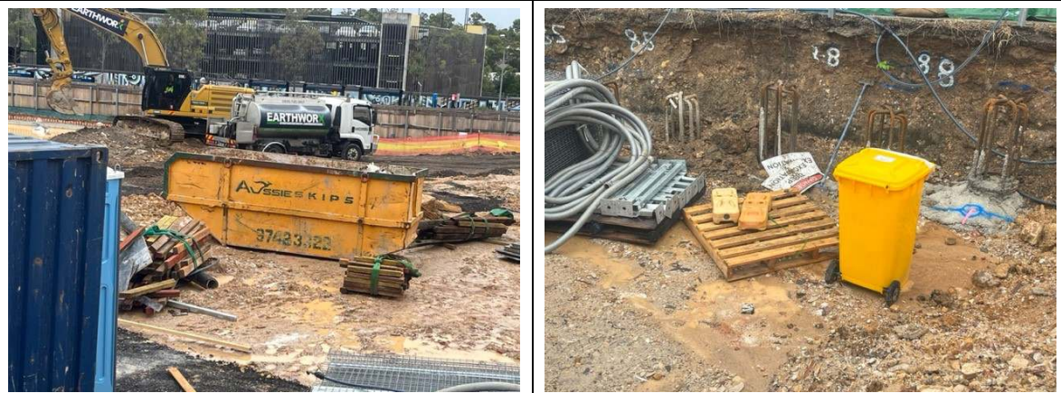
Photos 10&11: Spill kit and waste storage in place.
