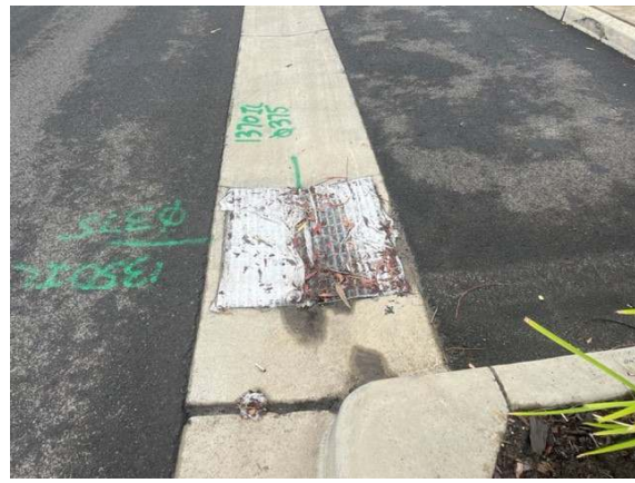
Photo 1: Drain protection in place on Andalusian Way
