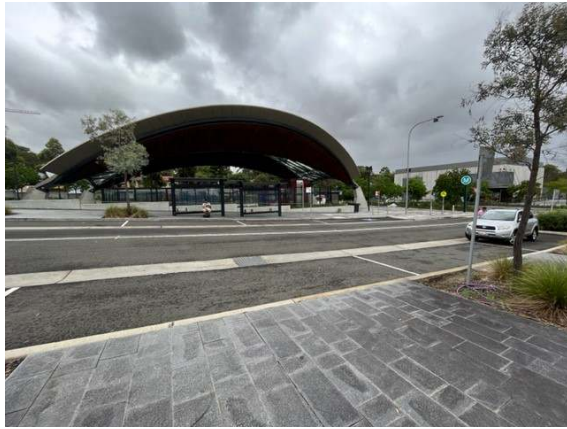
Photo 16: Neighbouring Castle Hill Showground Metro Station
