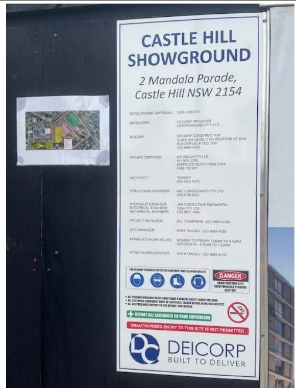
Photo 15: Compliant site notices were in place on the boundary hoarding at site accesses
