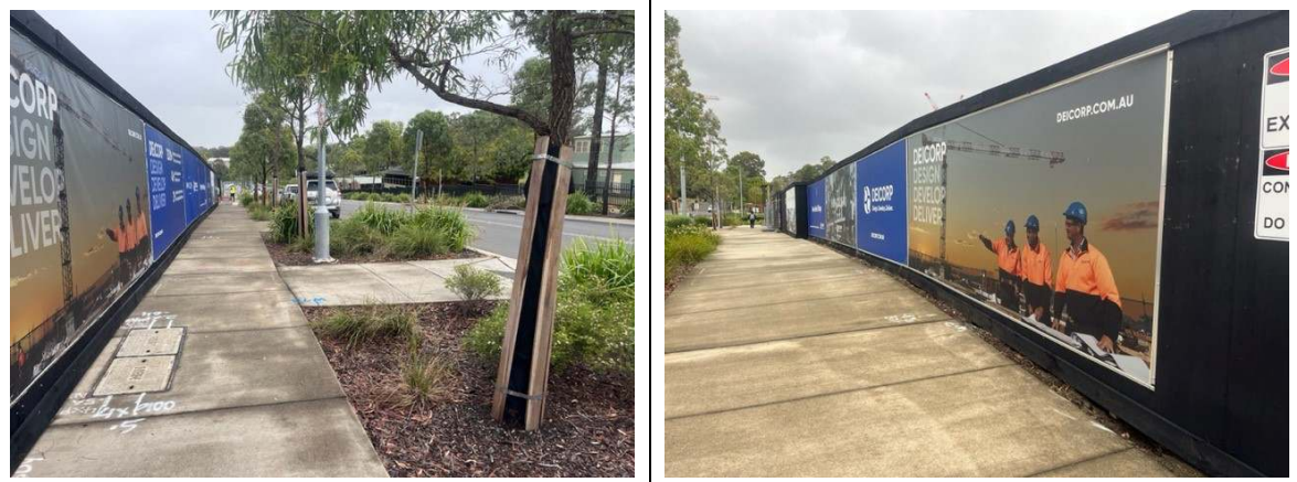
Photos 7&8: Hoarding in place along site boundaries. Tree protection in place on De Clambe Drive.
