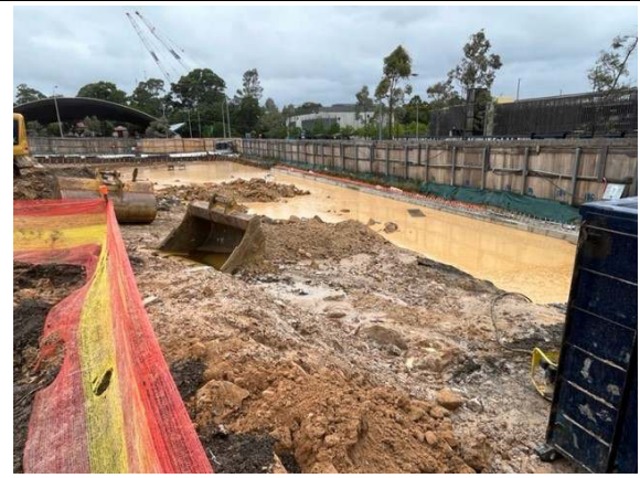
Photos 12&13: Water had accumulated in the SW corner of the site. A sediment settling tank was in place in preparation for dewatering.
