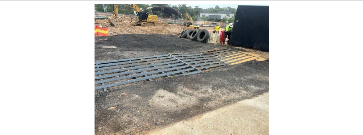
Photo 9: Shaker grid in place at heavy vehicle exit onto De Clambe Drive. No tracking observed.
