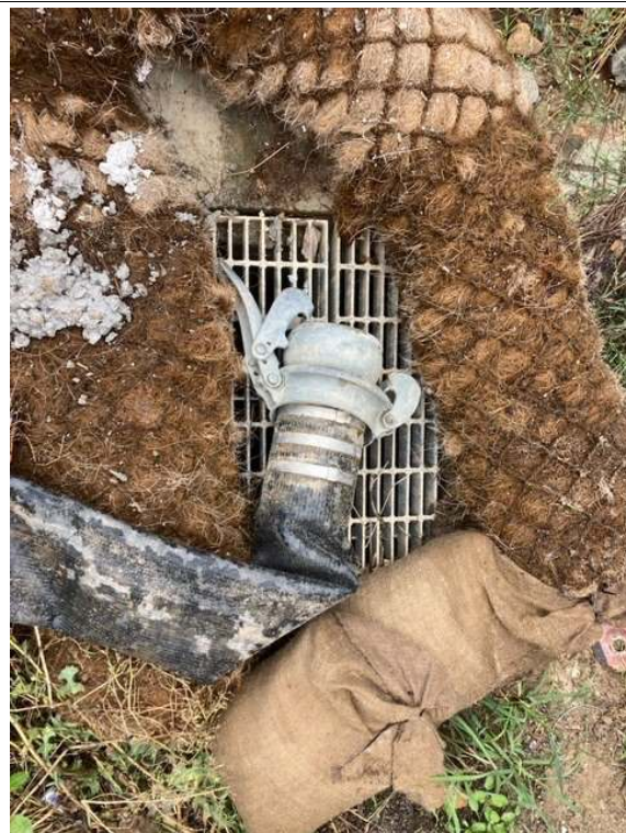
Photo 14: Controls were in place around the stormwater discharge point
