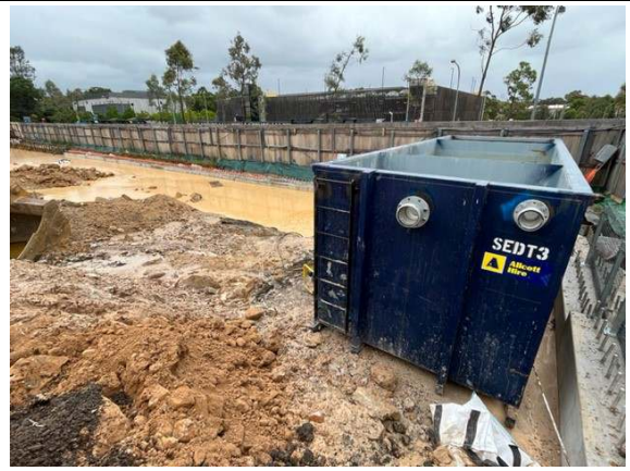
Photos 12&13: Water had accumulated in the SW corner of the site. A sediment settling tank was in place in preparation for dewatering.
