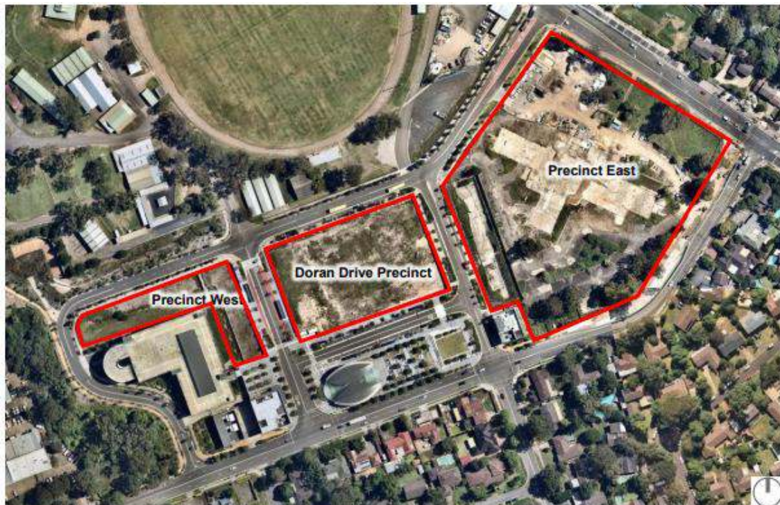
Figure 2: Doran Drive Precinct Site Location (centre) prior to development, Source: Nearmap 2022 / DPE Modification Assessment, 2022
